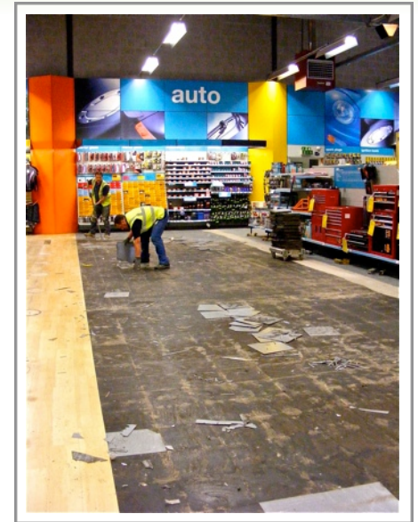
Hull Flooring's team collect the uplifted material
